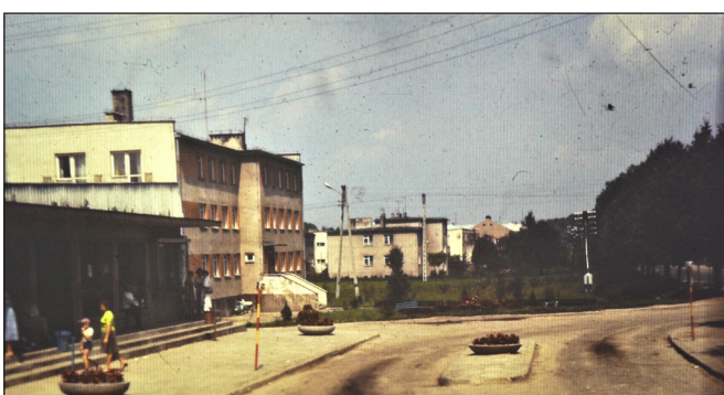
Bus station in Blazowa - 1980s
