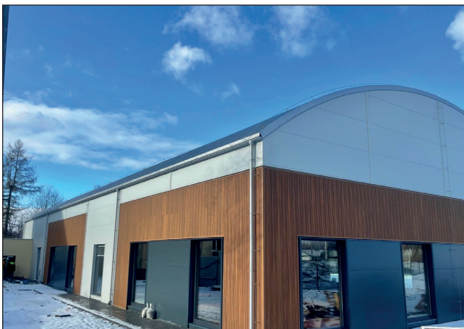
Under construction - sports hall at the Primary School in Nowy Borek.
