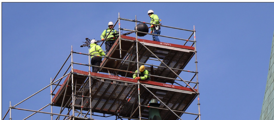
Renovation of the cross on one of the church's towers.
