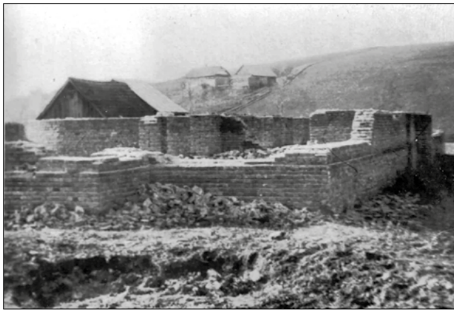
Construction of the Community House.
