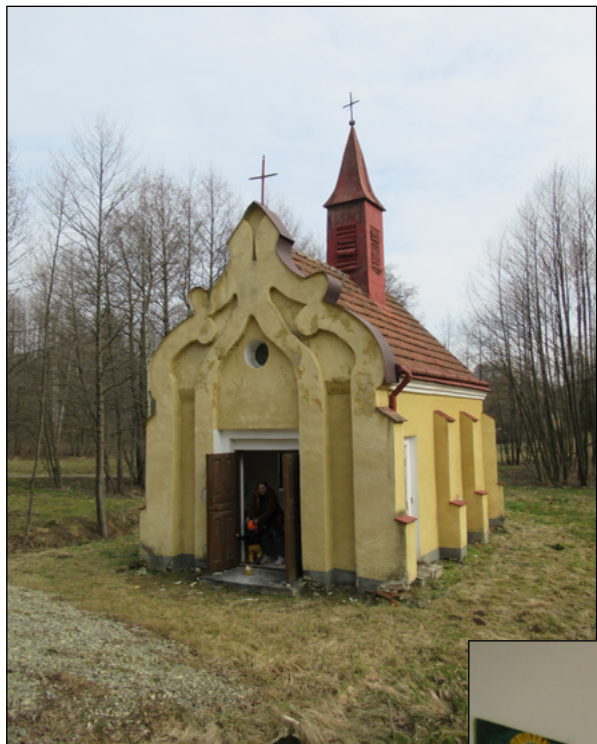
Chapel before renovation.
